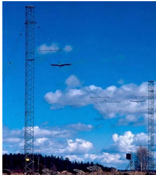
Bredbandsdipol 2 – 12 MHz 10 kW
